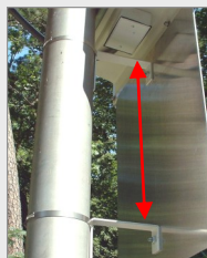
Installed extender brackets
