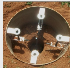
Installed concrete form with anchor bolts
